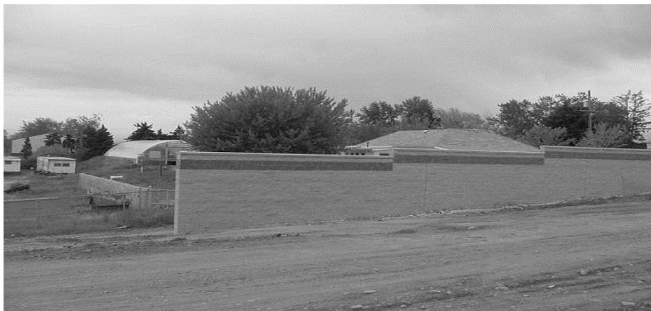
Illustration 18-1: Cast-in-Place Masonry I-76 East of York Street
